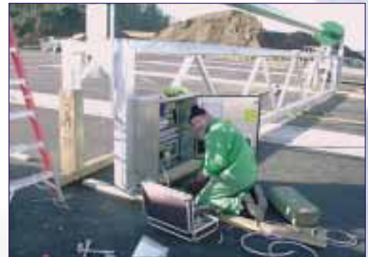
UTV composting plant in the U.S. - installation of mobile cover winding machine
