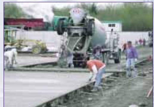
Concreting the site for a UTV composting plant in the U.S.
